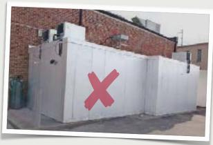
• Exposed exterior coolers are not allowed. Needs to blind with architecture or be screened.
