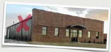
Masonry should wrap corners of the building to create more mass than a thin veneer.
